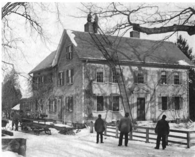
45 Men Repairing Damaged Chimney
